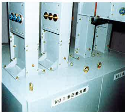
SWITCHBOARD CONNECTIONS (FLANGED ENDS)
